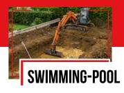
Digging to the exact dimensions and slope of the pool becomes child's play with the iDig guidance system.
